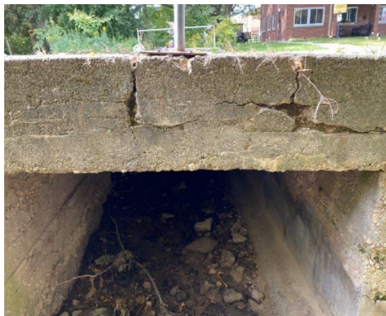
Dunke Culvert 2026 replacement project
